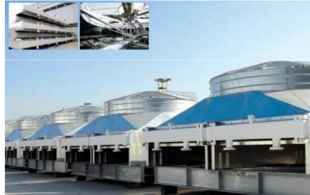
Air Cooled Heat Exchanger
