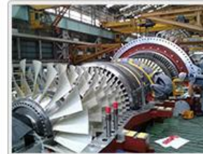
Blade Ring Assembly & Bolt Tightening
