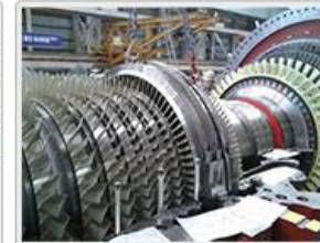
Blade Ring Assembly & Clearance Check
