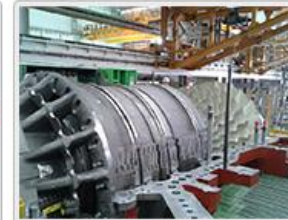
Blade Ring Dismantling, Lifting
